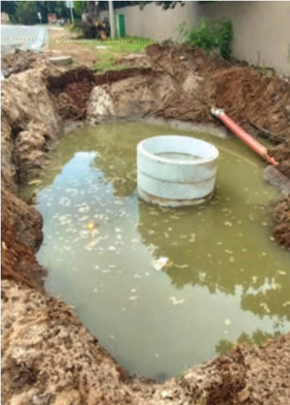
Sewage fills up a hole where it also flows into a damaged stormwater pipe, Arendskloof, 15 Feb 2023.
